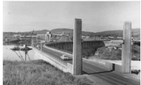
Jinja City Owen Falls Dam
