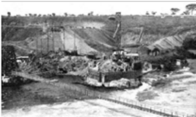
Construction of Owen Falls Dam in Jinja
